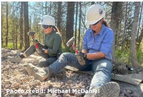
CDTC volunteers Dom and Mikaela (bffs from Iowa!) crush in gravel to make a level surface for a turnpike in Yellowstone National Park.
