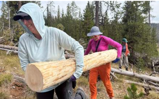
Volunteers carry a log to be used in construction of a step in Yellowstone National Park.
